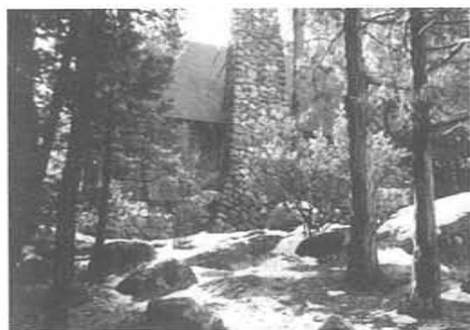
North end of house.
