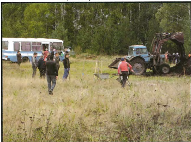
Digging and preparation of the site
